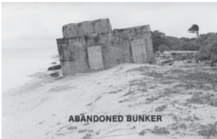
This was Station 77. The left door was the entrance to the timing and firing distribution station; the right door led to the telephone switchboard; and the structure on the roof (Station 1511) housed camera mounts. These were constructed for Operation Redwing (1956) on Runit Island, Enewetak Atoll. Shifting sands have caused this bunker to lean toward the water.
